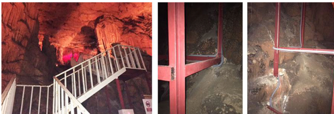
Fig. 7 Implementation details of metal constructions and electrification
