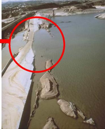
Figure 2.8. Lower San Fernando Dam after San Fernando Earthquake of 1971.
