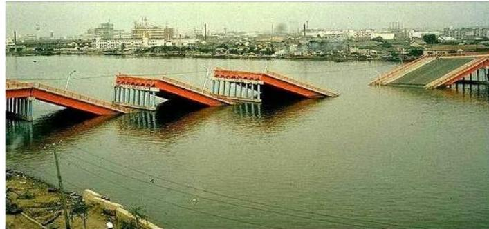
Figure 2.10. Lateral Spreading Problem After the 1964 Niigata Earthquake
