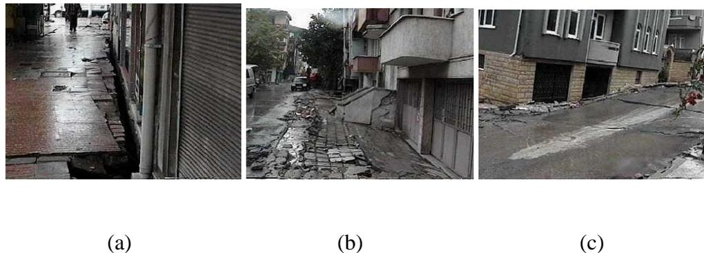
Figure 2.7. Examples of Settlement of Buildings after Marmara Earthquake, 1999
