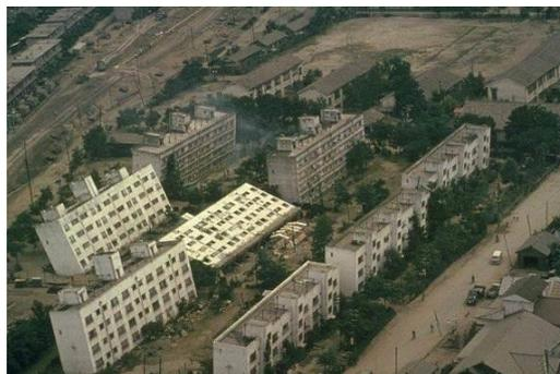
Figure 2.11. Bearing Capacity Problem After 1964 Niigata Earthquake
